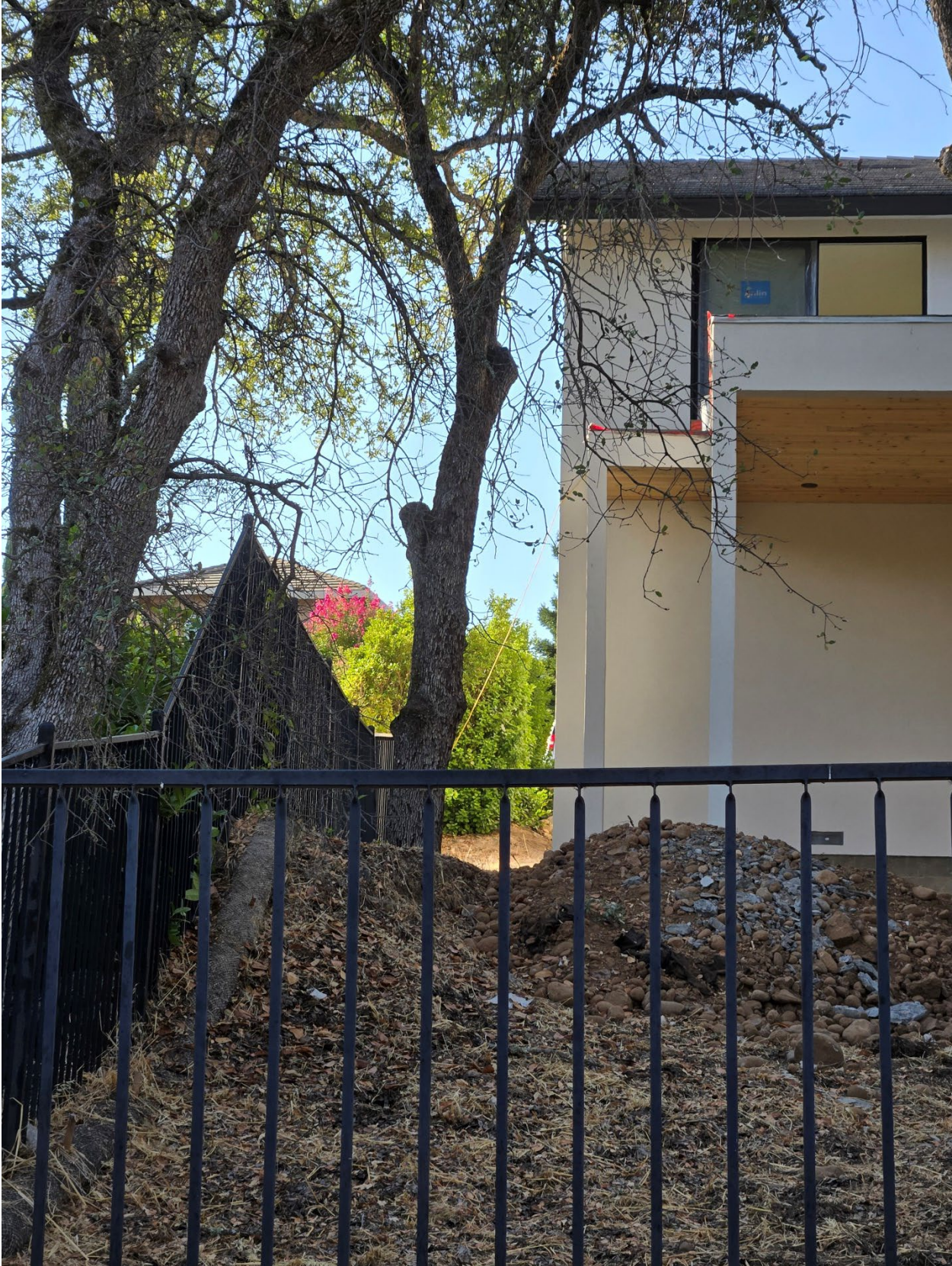
Figure 3 Saved Tree near New Home Construction View2
