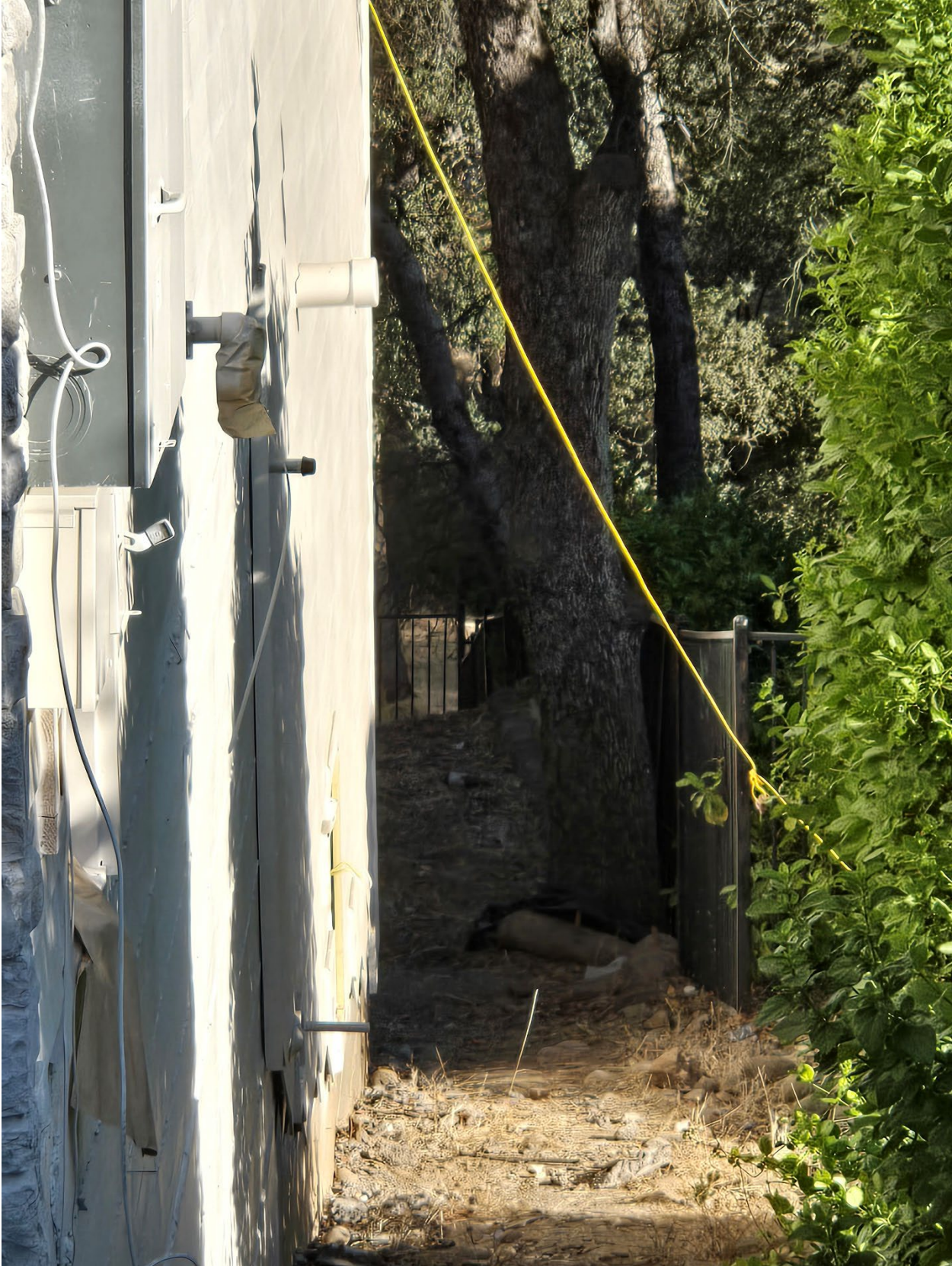
Figure 2 Saved Tree near New Home Construction View1
